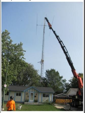
Once that was done, they used an angle grinder to cut the legs off the tower. They very carefully lifted the tower high up and over the roof of the house, around a street light, and onto the front street, where they lowered it to the street. Finally, they cut the tower up and loaded it onto a trailer for scrap. I was able to rescue the TailTwister rotator, before they left.
