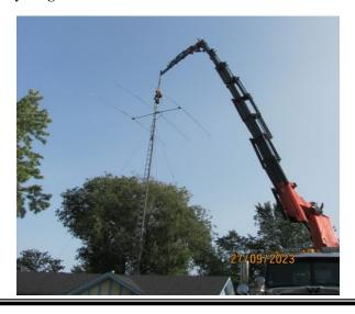
The truck had 3 axles in the back and 2 in front. They parked on the neighbour's driveway, The crane unwrapped, until the top was about 80 feet in the air. Their operator sat in a Bosun's Chair, and was raised above the antenna, then lowered enough to attach a cable to the tower. Next, their operator, who was a licenced arborist, cut away tree branches that were in the way of removing the tower.
