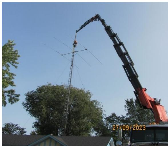
The truck had 3 axles in the back and 2 in front. They parked on the neighbour's driveway, The crane unwrapped, until the top was about 80 feet in the air. Their operator sat in a Bosun's Chair, and was raised above the antenna, then lowered enough to attach a cable to the tower. Next, their operator, who was a licensed arborist, cut away tree branches that were in the way of removing the tower.
