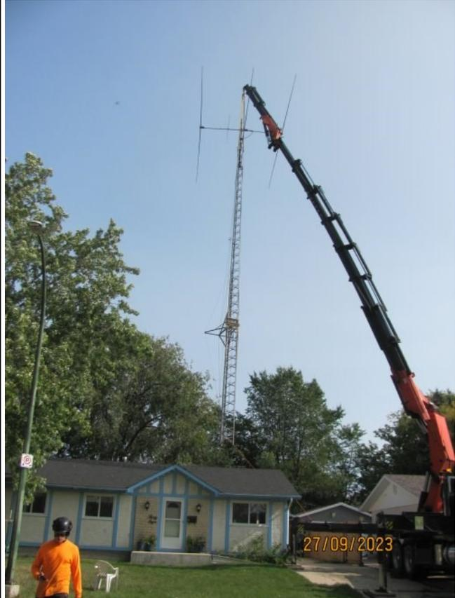
Once that was done, they used an angle grinder to cut the legs off the tower. They very carefully lifted the tower high up and over the roof of the house, around a street light, and onto the front street, where they lowered it to the street. Finally, they cut the tower up and loaded it onto a trailer for scrap. I was able to rescue the TailTwister rotator, before they left.
