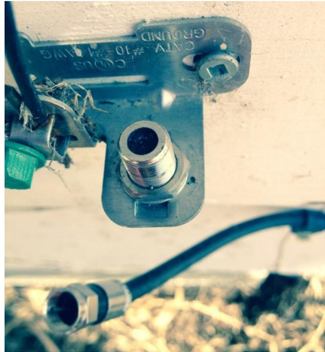
After replacing the bulkhead connector and the terminations from my stash of parts here at the house, mounted the ground block horizontally so that the connections don't fill up, and put a drip loop and linerless rubber splicing tape on it as well. I had to shorten the cable a bit to do this, so it doesn't follow the siding on the house now and looks a bit odd ... oh, well.
